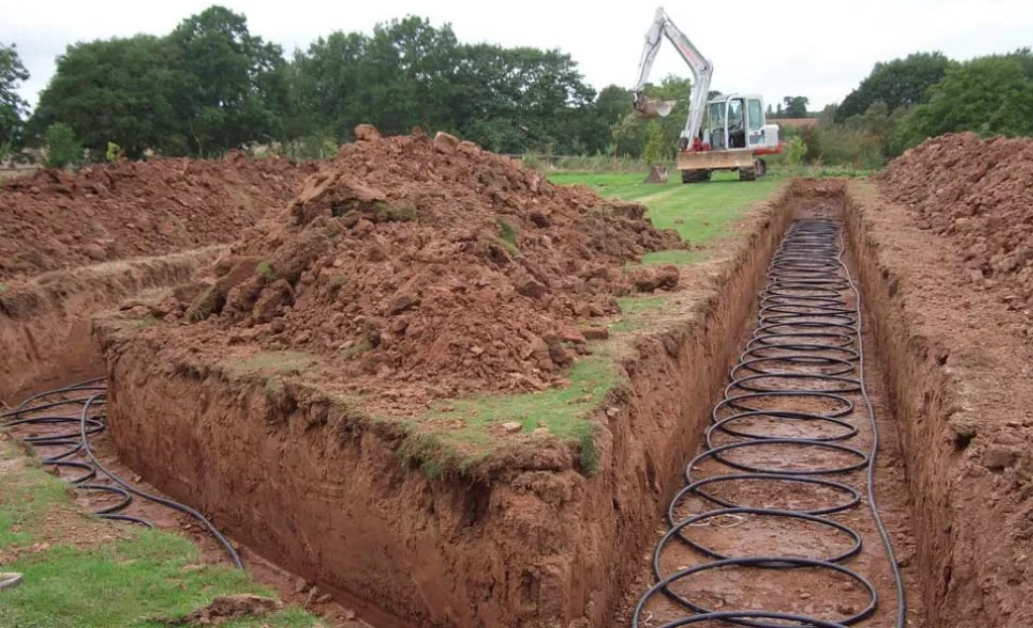
Horizontal slinkies seen inside a trench (Image credit: Kensa Heat Pumps)
