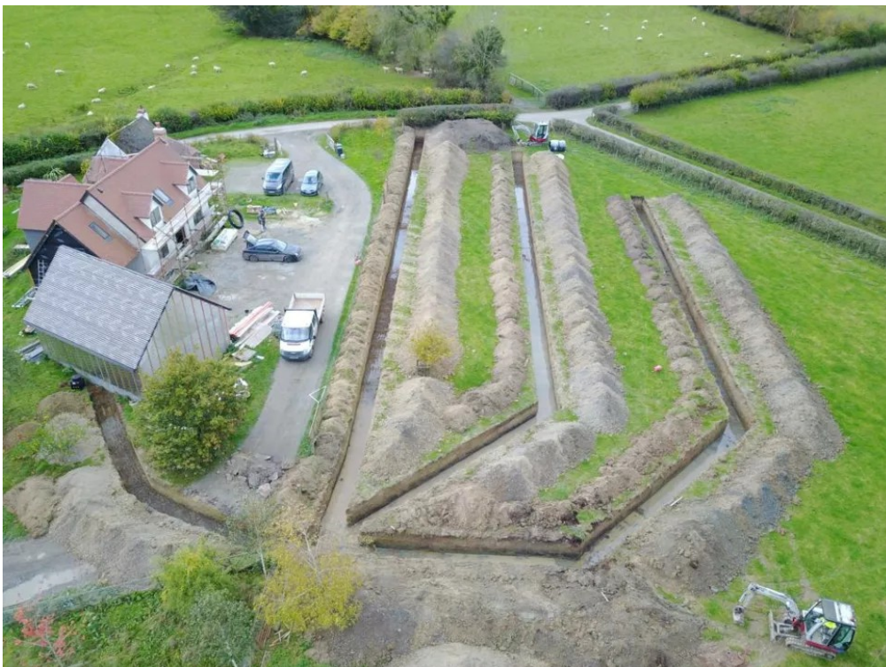
Horizontal slinkies seen inside a trench (Image credit: Kensa Heat Pumps)
